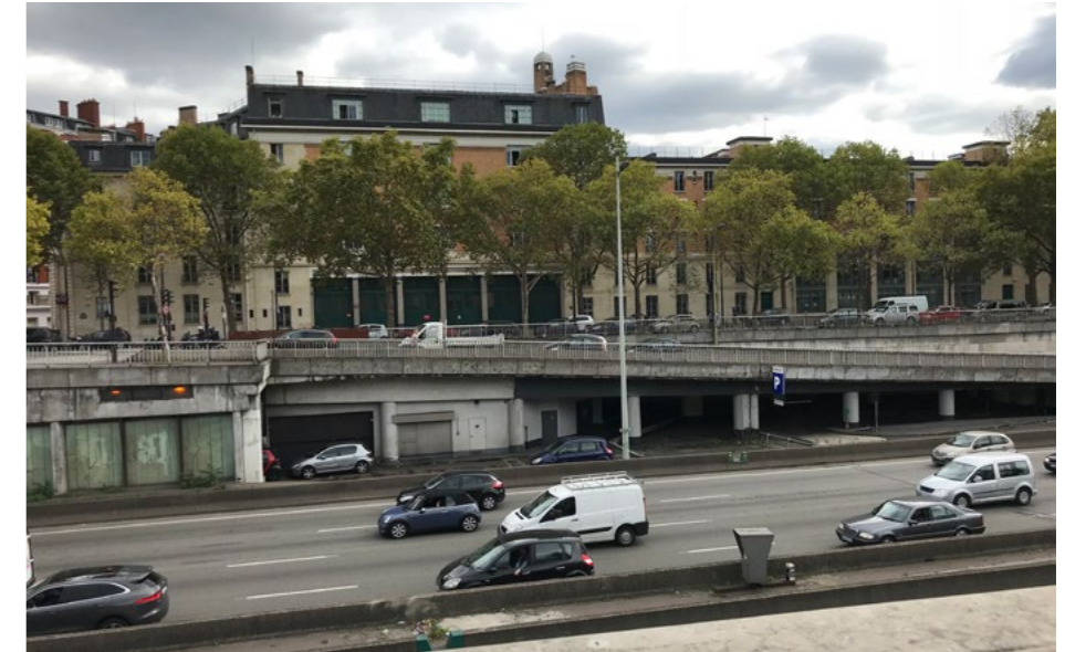
Figure 8 - Former petrol station at the Porte de Champerret, which is the subject of a project to convert it into a logistics site (Paris 17th arrondissement). ©Sogaris
